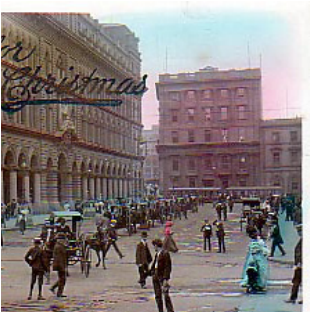
Figure 9_ Martin Place_ State Library NSW
