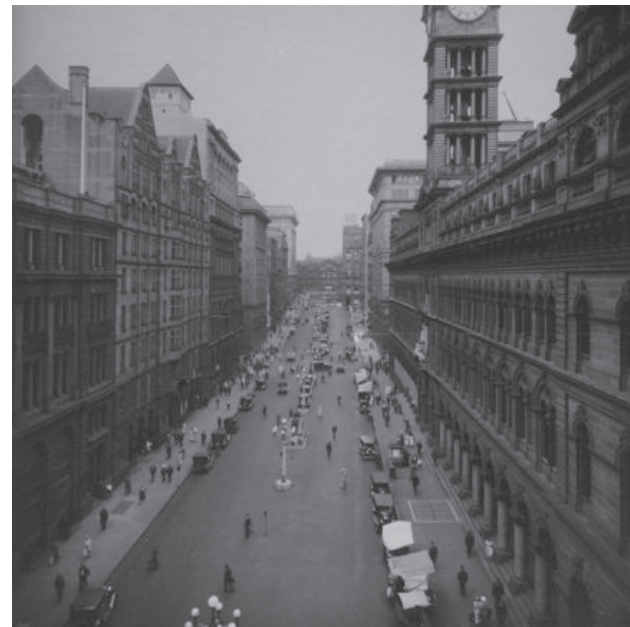
Figure 11_ Martin Place_ State Library NSW
