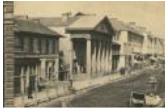
Figure 3_ Original Post Office on George Street
